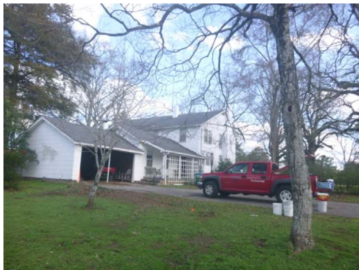
Figure 6. Back of the ca. 1834 house showing the rear addition and garage.
